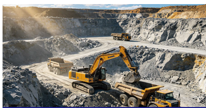
Large-scale Earthworks & Engineering Surveying
