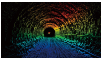
Underground & Enclosed Spaces
